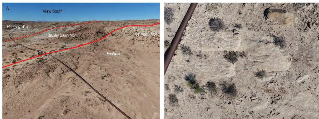
Figure 17. Left: Perspective view looking south where the red trace is the fault crossed by the pipeline. Brann Johnson is at the fault contact crossed by the pipeline for scale. Right: Drone image looking down at a zone of deformation bands in the Salt Wash sandstone at the location of Brann Johnson in the left figure. The pipeline is in the upper left. Drone photos by Rex Cole.
